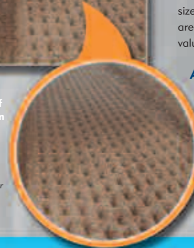
Aqueeled surface Increased percolation of water and vast reduction in run-off
